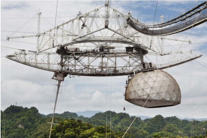
Figure 2. Arecibo Observatory 2-dof Azimuth Arm www.gravitec.com
